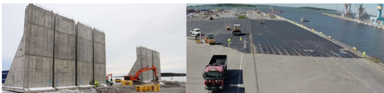
Picture 27 New quay walls for the new container berth in Port of Rauma, waiting to be installed and on the right, the completed quay. The height of elements is 15 meters. Source: Konepörssi/Rauman Satama Ltd. https://www.koneporssi.com/uutiset/lisaa-satamalaituria-raumalla/
